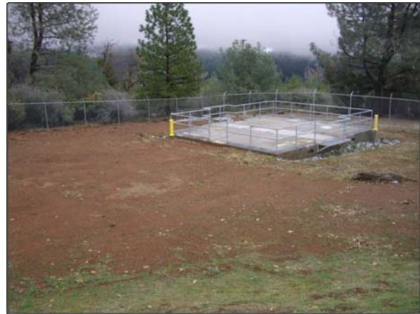
Photo 8 – Existing Pressure Reducing Station at Reservoir B
