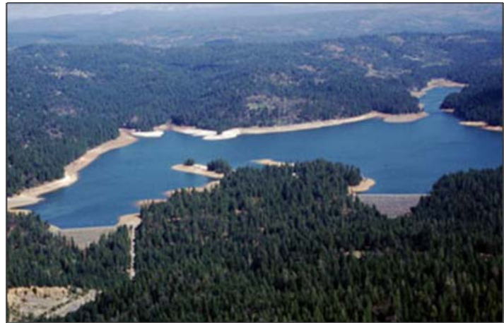
Photo 7 – Sly Park Dam, Hydroelectric Project at Dam Section on Right
