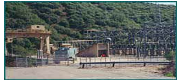
White Rock Powerhouse
